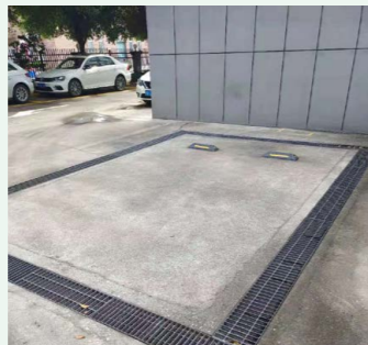
Sewage pipe network in the car wash zone
